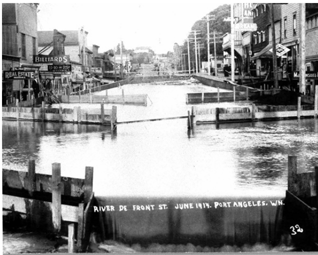
Figure A.04 – Downtown Port Angeles was dramatically transformed in 1914 when street-level grades were raised 12 feet or more following a massive sluice operation - effectively a man-made mud slide using a nearby hillside for source material.
