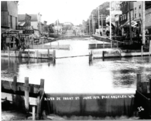
Figure A.04 – Downtown Port Angeles was dramatically transformed in 1914 when street-level grades were raised 12 feet or more following a massive sluice operation - effectively a man-made mud slide using a nearby hillside for source material.
