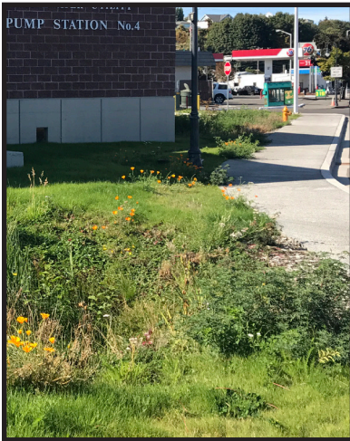
Rain garden and pervious concrete at new City pump station.
