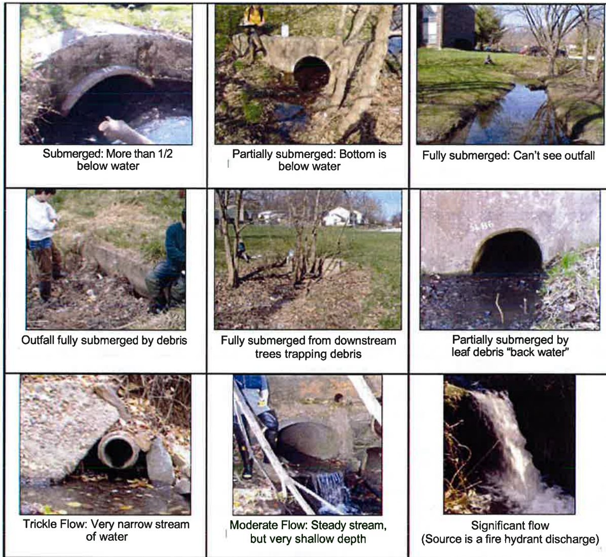
Figure 8.4.1: Characterizing Submersion and Flow
