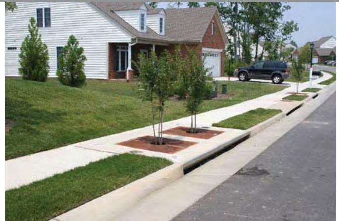
FILTERRA UNITS EXAMPLE
