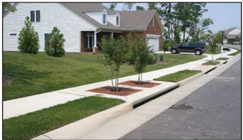
FILTERRA UNITS (EXAMPLE)
