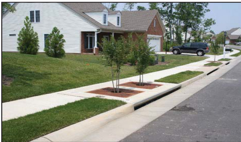
FILTERRA UNITS (EXAMPLE)
