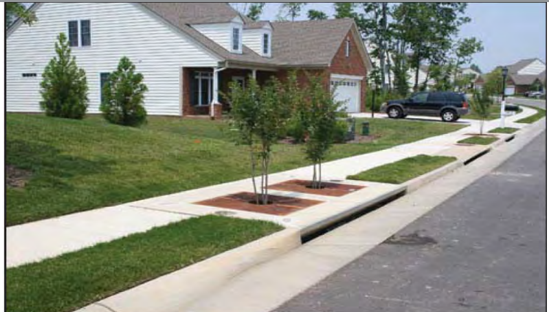
FILTERRA UNITS (EXAMPLE)
