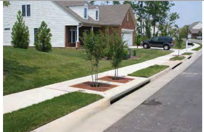
FILTERRA UNITS EXAMPLE
